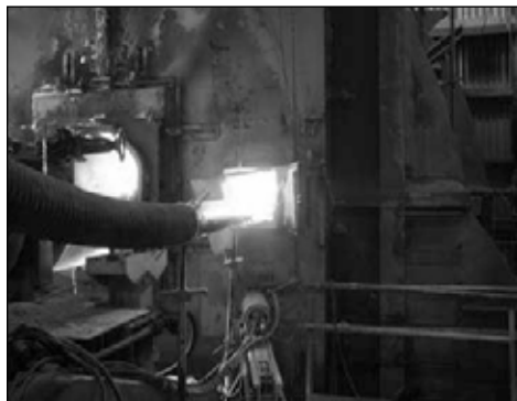
Figure 1: Biomass fuel mixture is delivered through the pipe on right side and the coal mixture on the left side of this picture.
